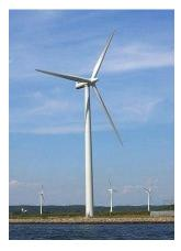
Harnessing the kinetic energy of wind can provide a renewable source of on-site electricity generation. Wind turbines need to be positioned where a frequent and steady source of wind is available that is not too turbulent or uneven in direction. Typically, wind turbines are positioned on the roof of buildings that are significantly higher than their surroundings and or located in open areas where there is minimum disruption to prevailing winds.
